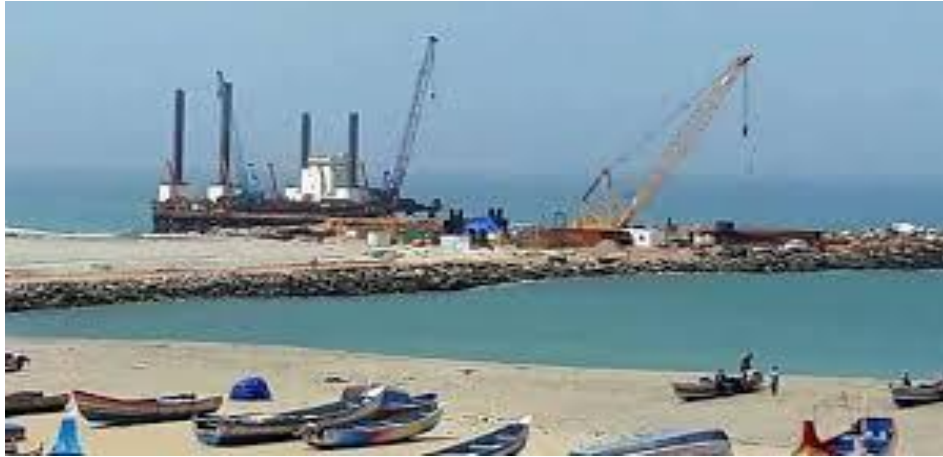
Figure 4.2.1 Project location photographs
