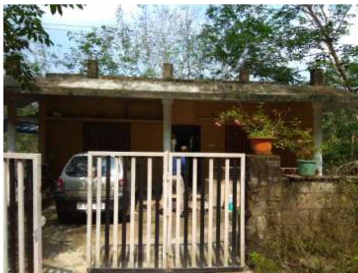
One of the Affected House
